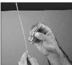
1. Wrap galvanized wire rope around an overhead building structural member
